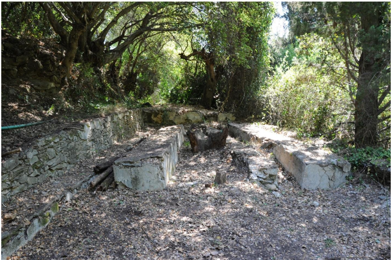
The “picnic area” at the Manganou spring, after being cleared in 2011
