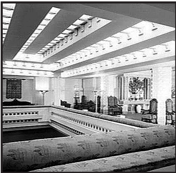
The void and ceiling above original stalls 1924
