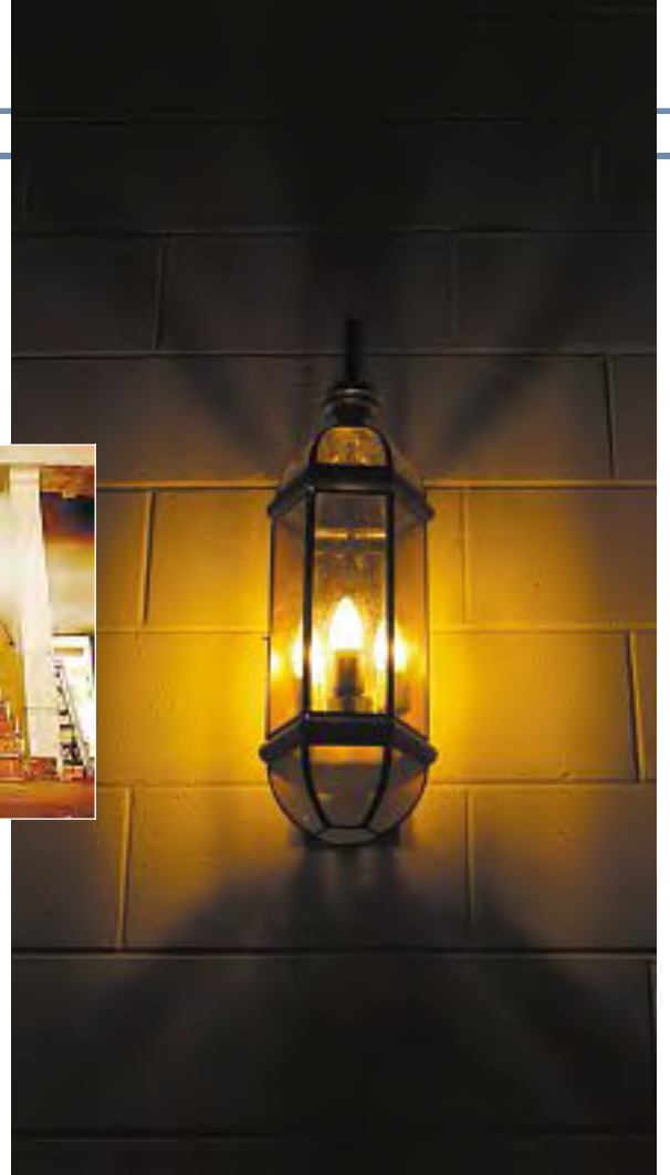
One of the newly installed heritage style lights at the Saraton Theatre.
