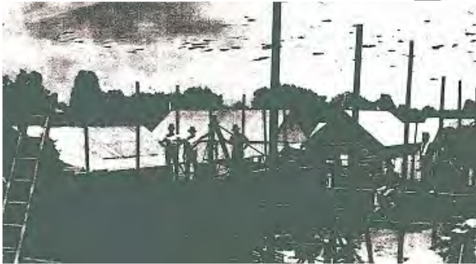
ABOVE LEFT: Construction of Saraton circa 1925. There weren't any cranes available so they used the same technology as building the 2500-year-old Parthenon in Athens. Two large posts acted as an A-frame crane to lift the large 18m (54ft) main balcony girder. ABOVE RIGHT: Anthony centre, Jack right and a cousin, Emmanuel, on the left, celebrating Australia Day circa 1912.
