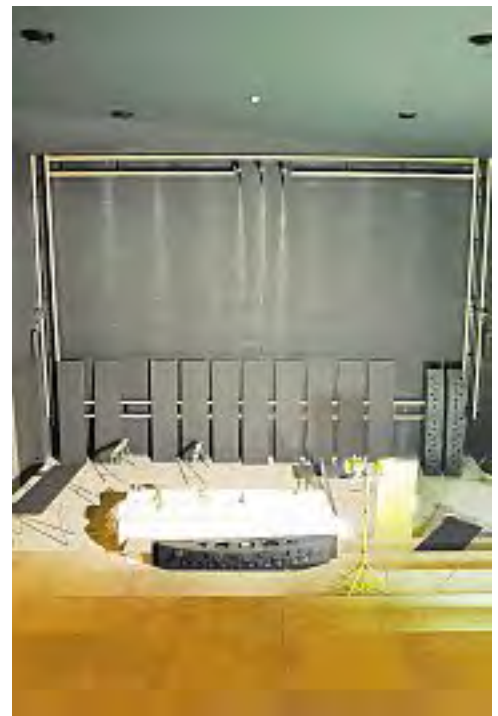
One of the new cinemas under construction at the Saraton Theatre complex.
