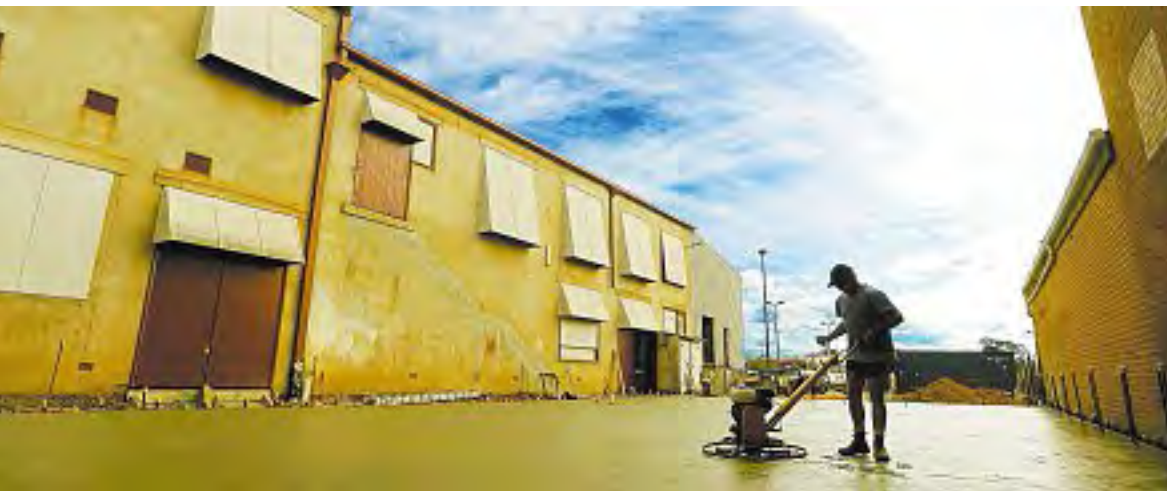
Builder Robert Wilson works on the newly-laid concrete slab for the additional theatres at the rear of the Saraton site.
