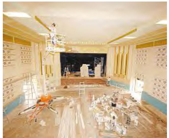
Paint contractor Bruce Bowling puts an extra coat on the facade of the Saraton Theatre ceiling. Work on the heritage building is continuing.
